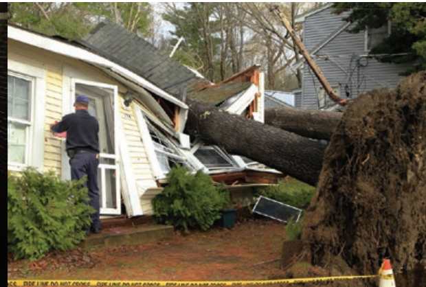
Overturned trees crushed this home.
